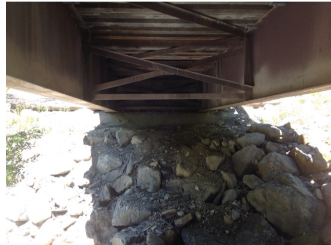
Right Bank Abutment when facing downstream
