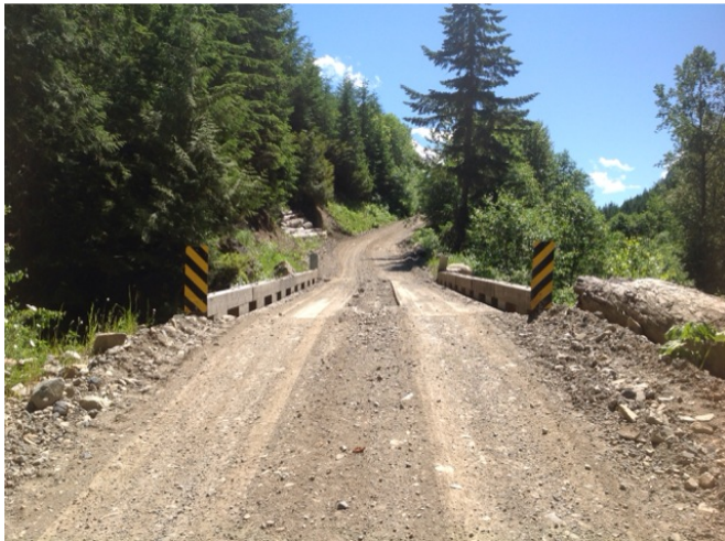
Approach from Right Bank when facing downstream
