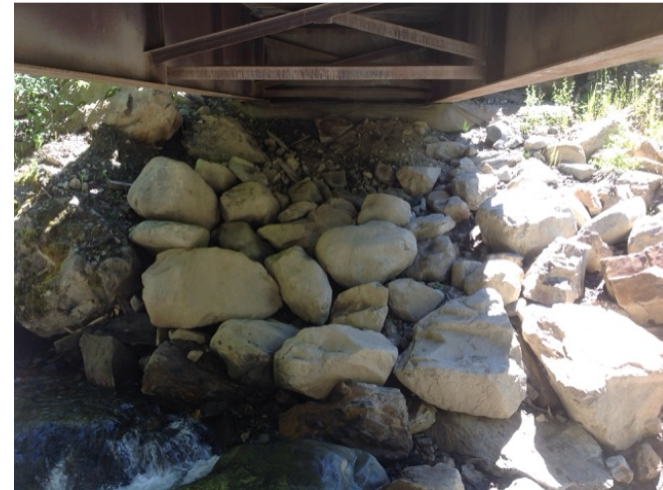
Left Bank Abutment when facing downstream
