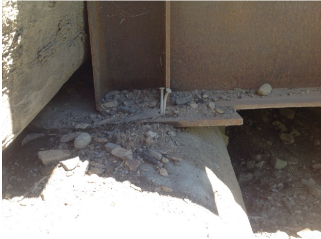
right down stream bearing
